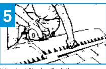
Nail each additional section in the same manner until entire ridge is covered. A chalk line may be utilized to ensure vent alignment. Cut last piece to length and install with original uncut end to the outside.
