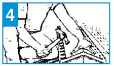
For appearance (to blend with the roof line), it is recommended that the **TruRidge™** vent be installed the entire length of the ridge. Position the first piece at one end of the ridge. Using 2-1/2" nails, for 3/4" deck penetration or penetration through the deck, which ever is less, anchor vent through preformed nail holes.
