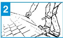
Snap chalk line on both sides of the ridge and no more than .750 (3/4) of an inch from the peak. **Note:** If a ridgepole is present, cut a wider gap to allow a minimum of  $1/2^{"}$  air gap on both sides of the pole into the attic space - but do not remove more than 2-1/4" of roof sheathing material from either side of the ridge.
